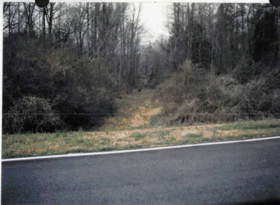
Sewer line off of Highview Road which runs north from Dairy Ridge Road (Grenade found here) J-41
