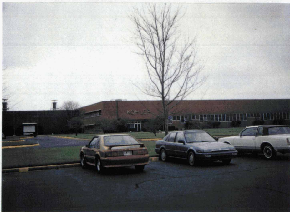
Kohler, Administrative Offices, located to the East of former Camp Croft cantonment area J-43
