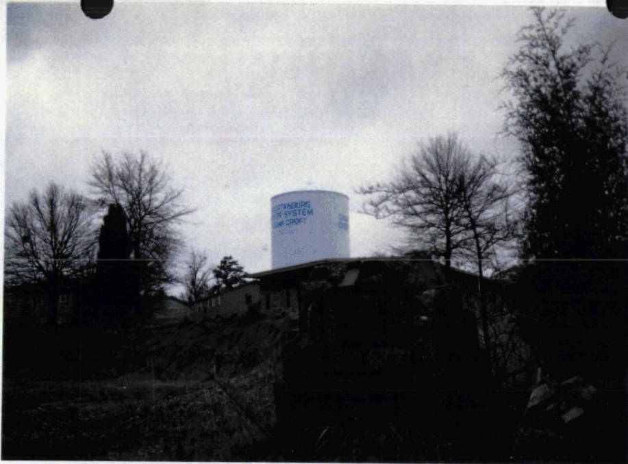
Water Reservoir, former Camp Croft and cantonment area stone markers
