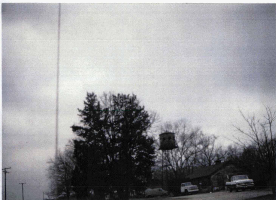
Training Range Tower just north of Dairy Ridge Rd J-12
