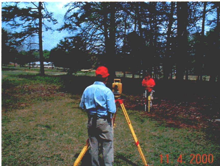
Figure 3: Surveyor and UXO Technician Using Electronic Total Station, Prism, and Schonstedt Locator to Stake Anomalies
