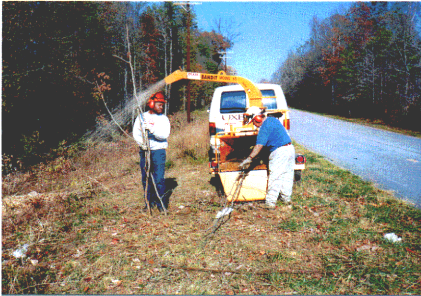
Figure 5: Chipping of Removed Vegetation
