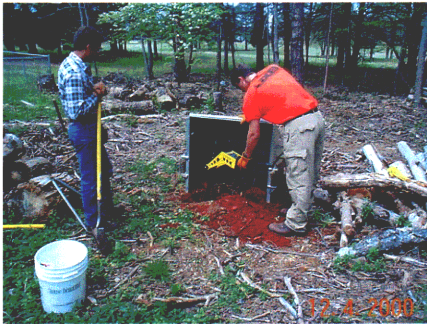
Figure 13: Miniature Open Front Barricade Used During Excavation
