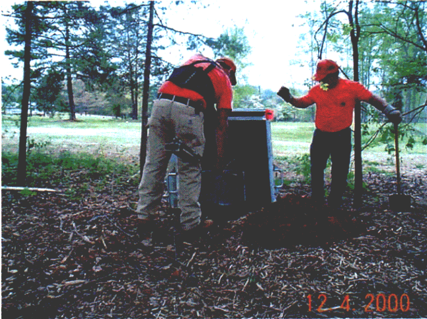
Figure 12: Excavation Utilizing Miniature Open Front Barricade
