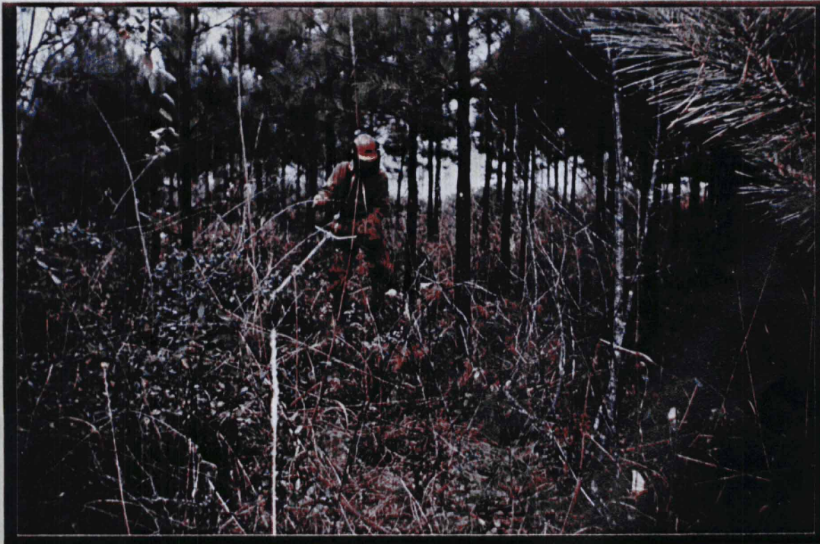
Grubbing and clearing of expanded landfill area, December 1994.
