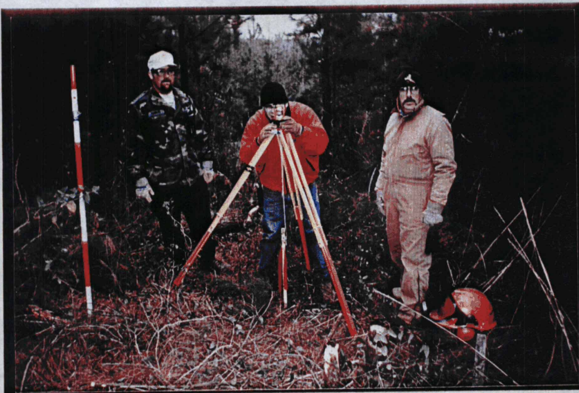
HFA personnel laying out grids in expanded landfill area, December 1994.
