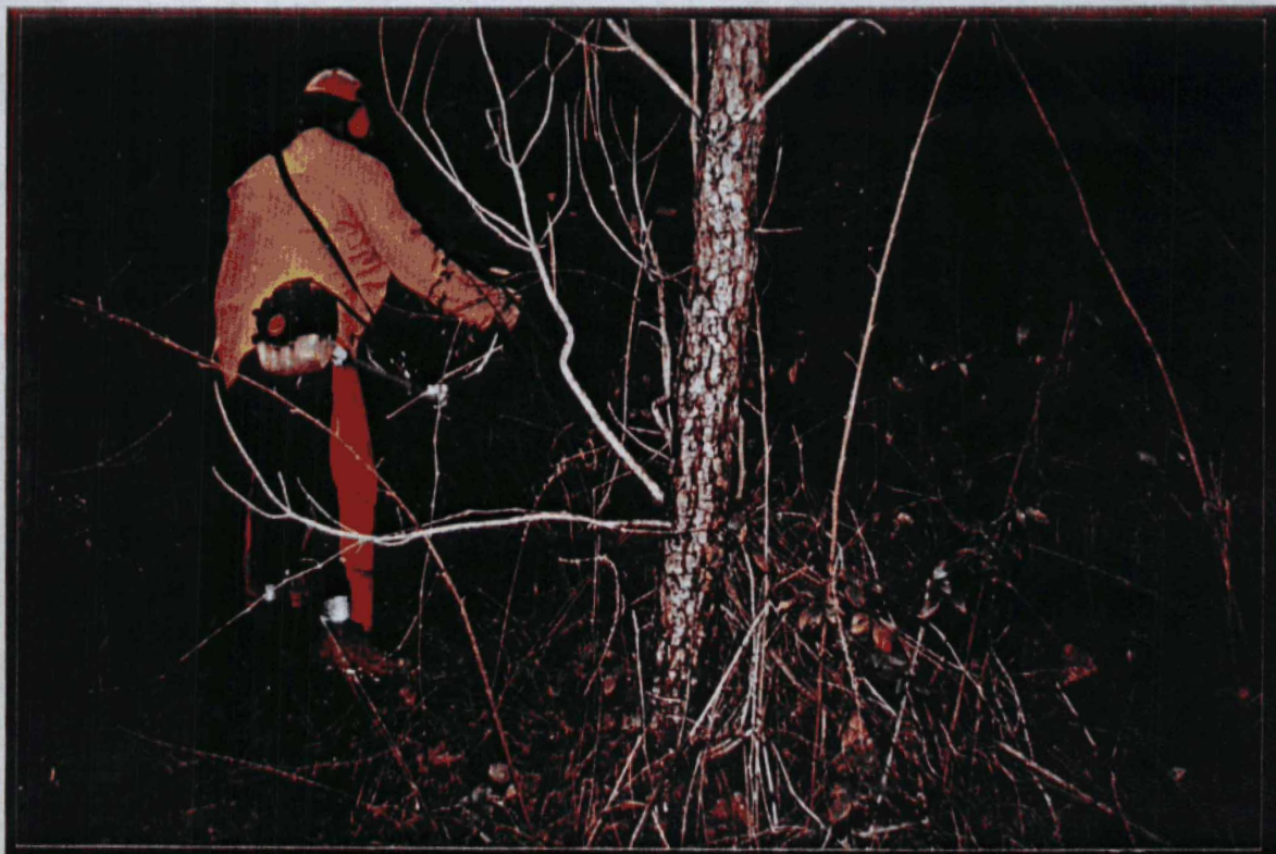
Grubbing and clearing operations.
