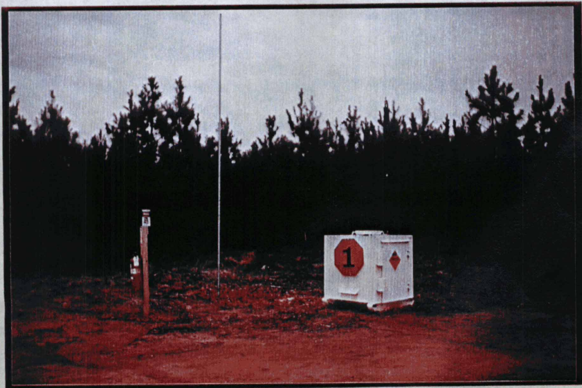
Magazine storage area, with lightning arrester in background.
